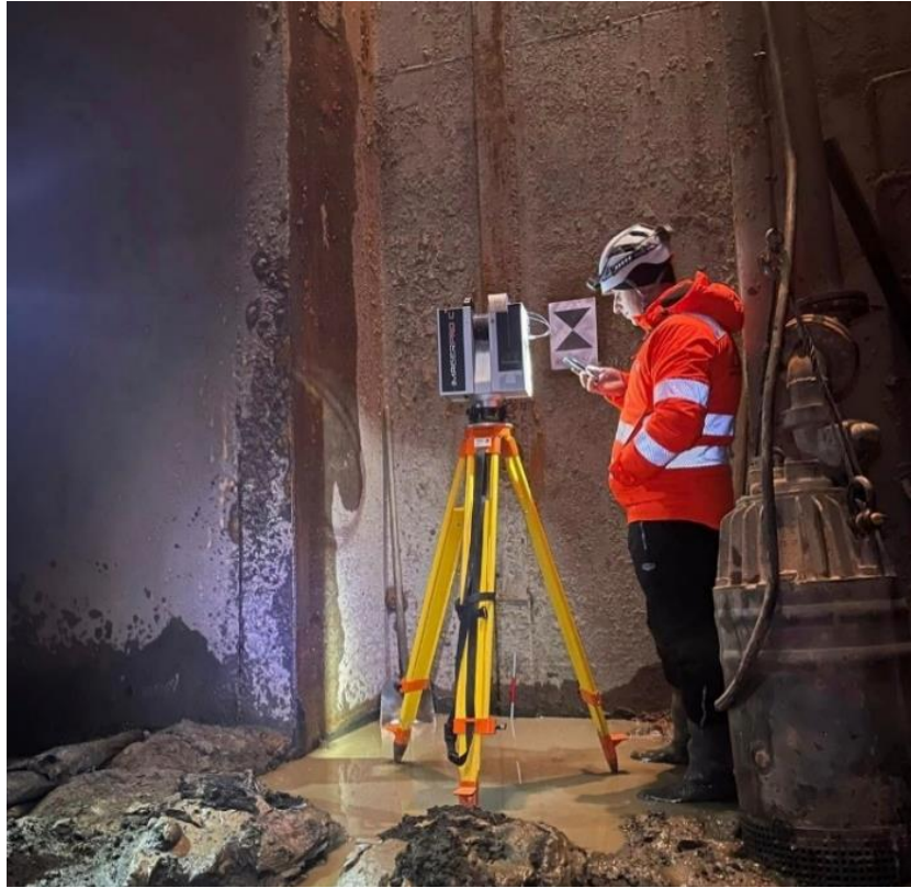
Fig. 4. Scan performed inside the valve
