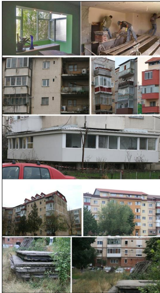
Fig. 1. Problems regarding the building blocks in Timisoara.
