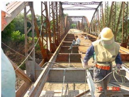
Sand blasting of the structure
