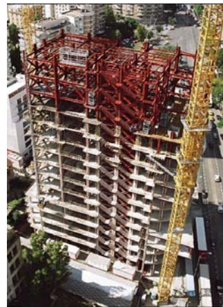
Fig. 2 The Bucharest Tower Center building in construction
