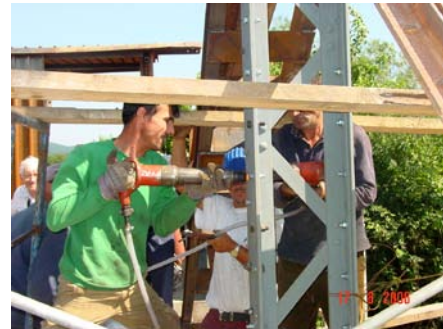
Riveting of the new strengthening steel elements
