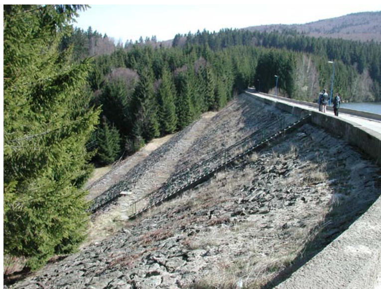
Studies regarding the dams safety running
